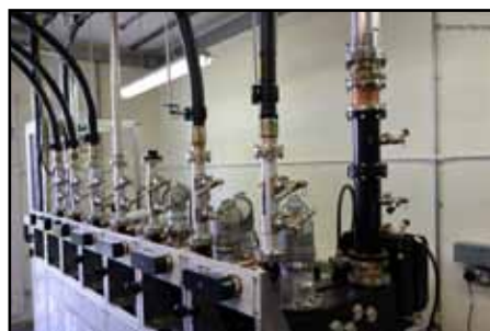
Output to the transmitters on the mast
